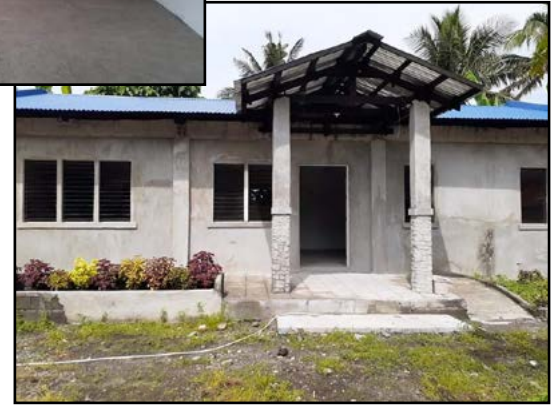
New church building
