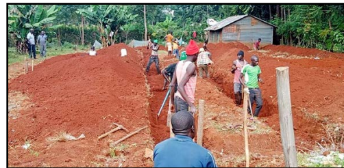
Digging the foundations
