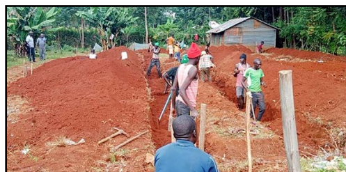
Digging the foundations
