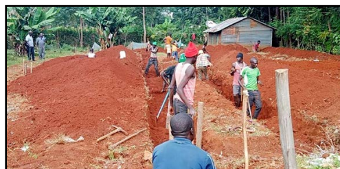
Digging the foundations
