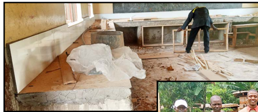
Work starting on the new laboratory
