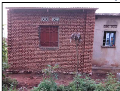
New storge building
