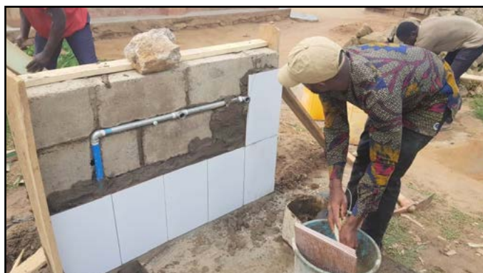
Building one of the water fountains
