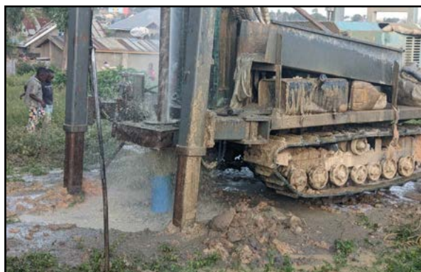
Drilling the borehole
