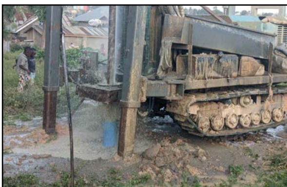
Drilling the borehole
