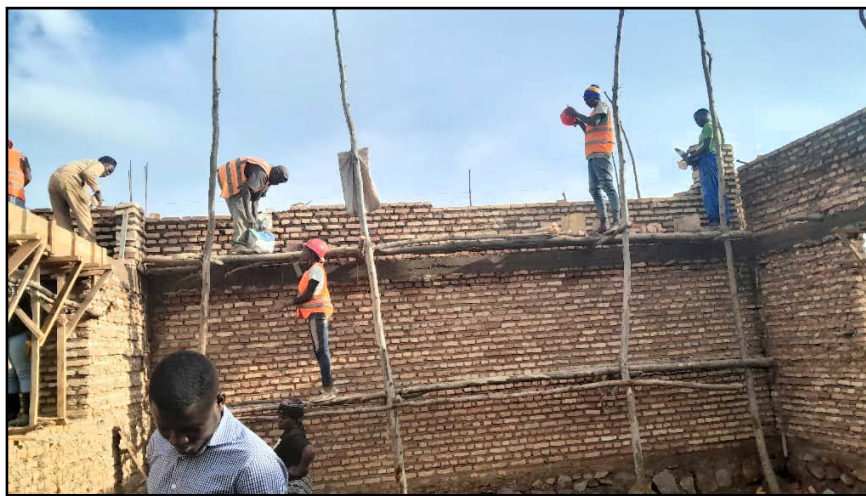
New Bible College construction
