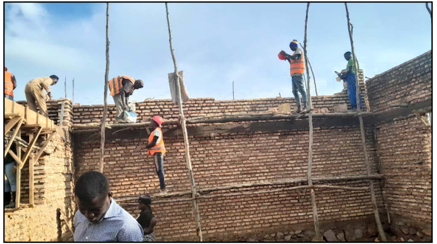
New Bible College construction
