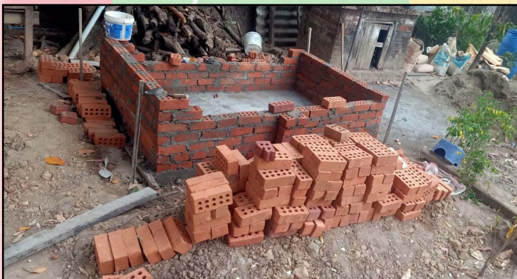
Baptismal pool being built in Yangon
