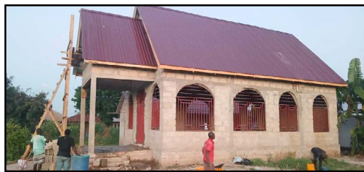
Morogoro church nearly completed.
